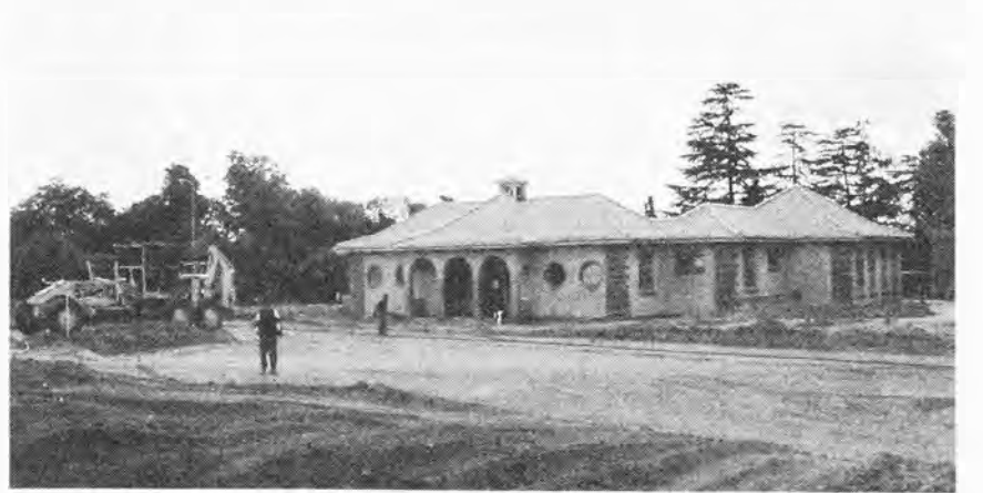
The new pre-school nearing completion, 27 November 1997
