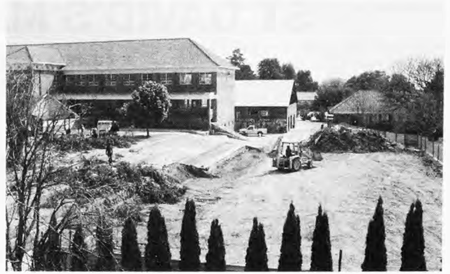
The site is cleared, 1 August 1997
