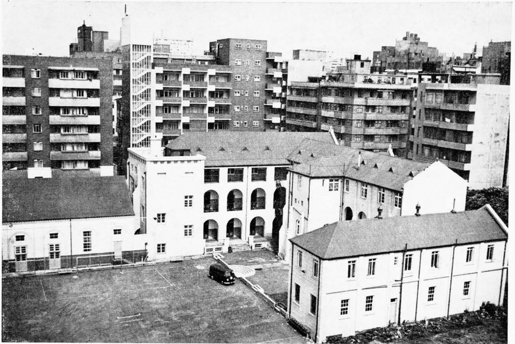
Present Koch Street School now hemmed in by modern city developments.
