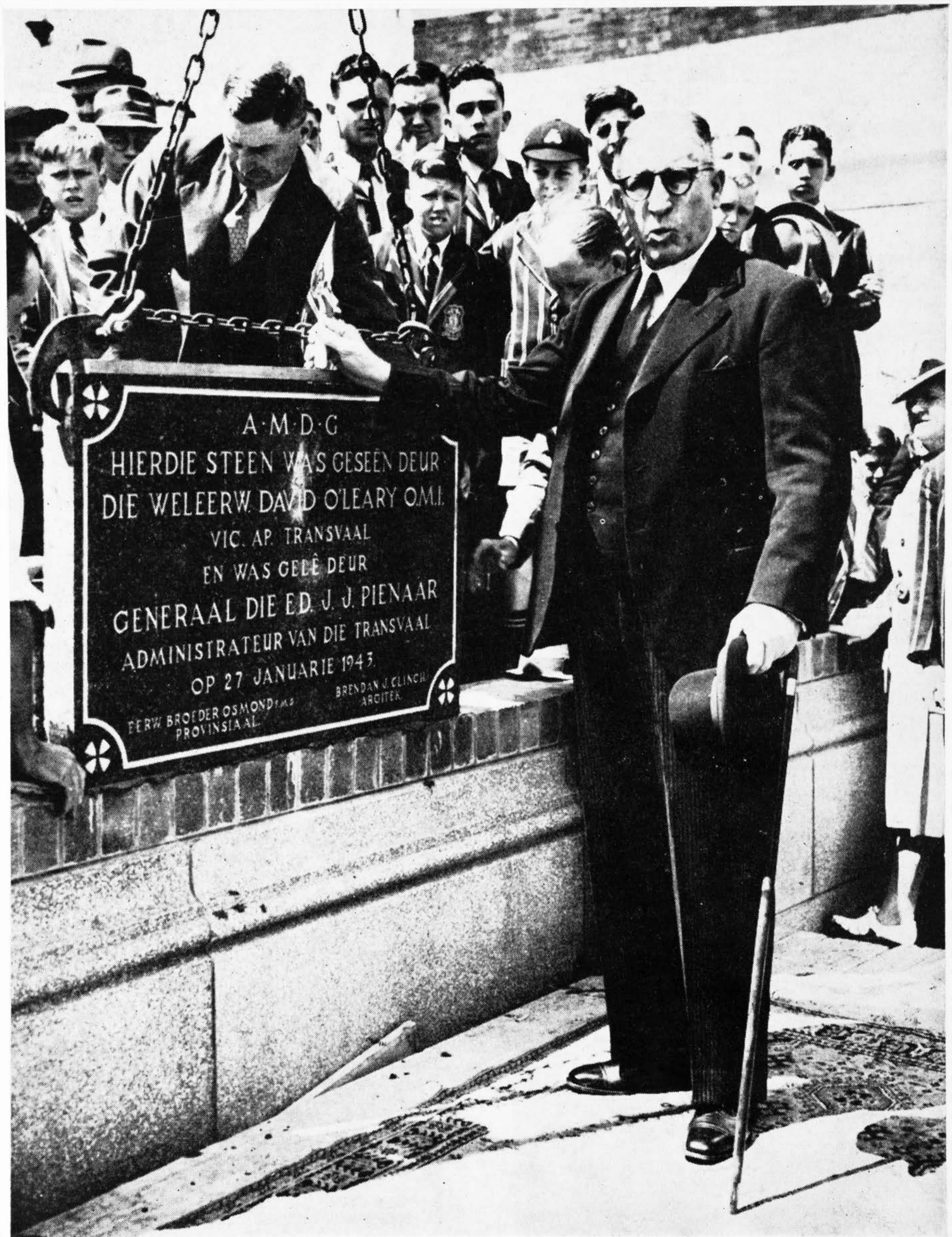
General J. J. Pienaar, Administrator of the Transvaal, laying the foundation stone, January 27th, 1943.
