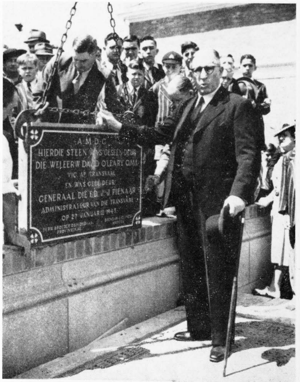
Laying of the Foundation Stone at Inanda by General J. J. Pienaar, Administrator of the Transvaal.
